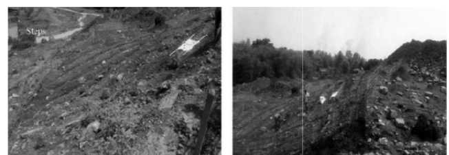
Figure 1 Preparation of Vetiver plantation site.
